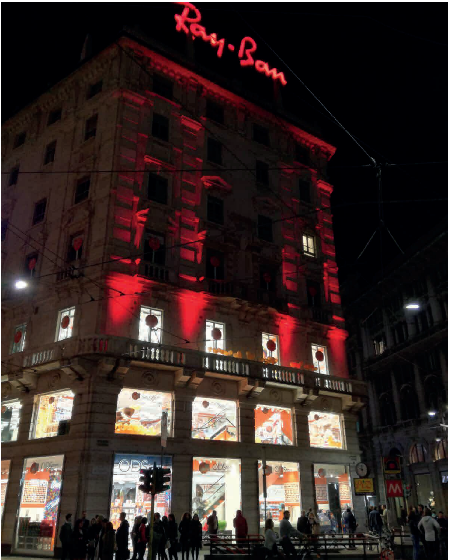
Architectural Outdoor - ODS Store, Milan, Italy
