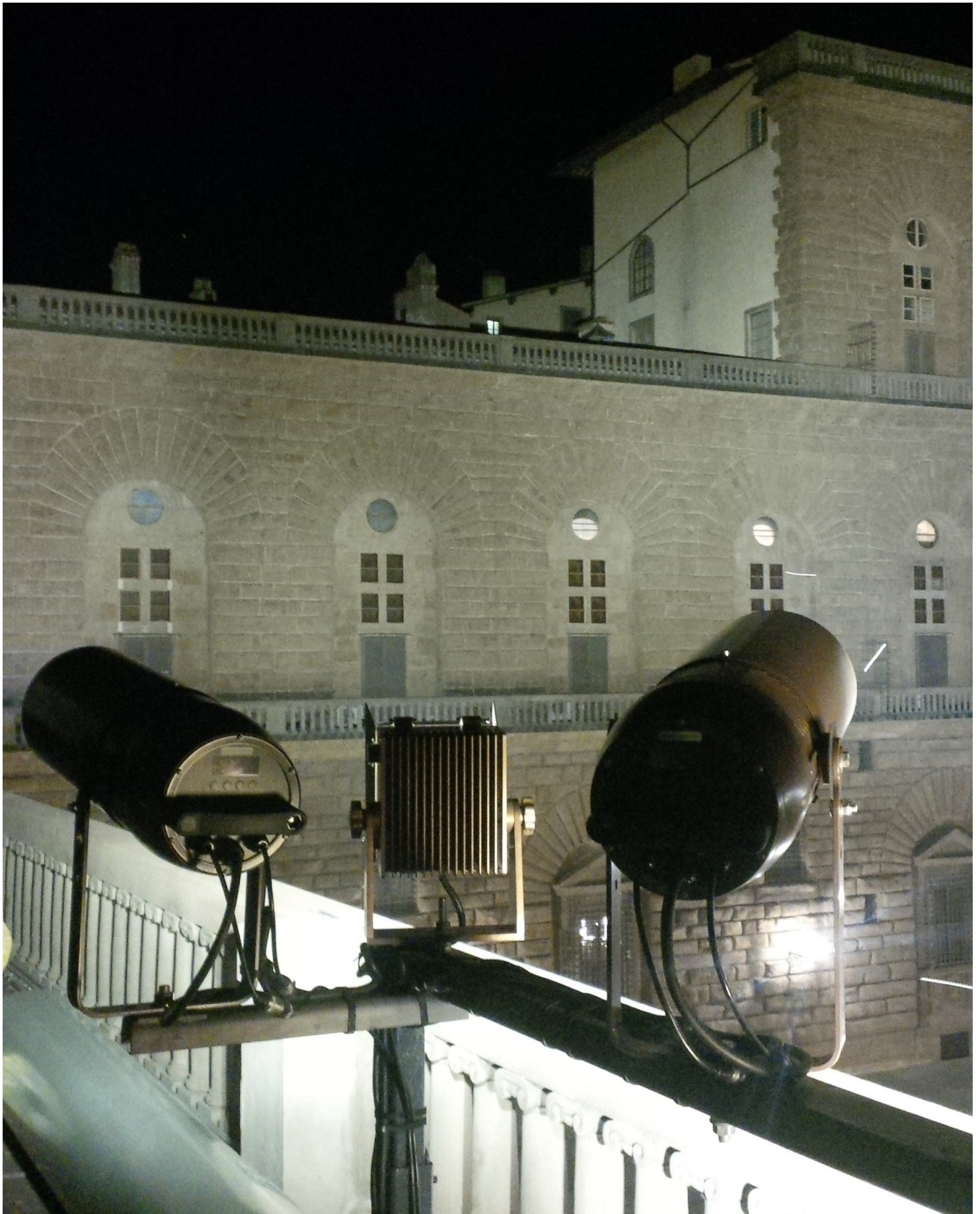
Architectural Outdoor - Pitti Palace, Florence, Italy
