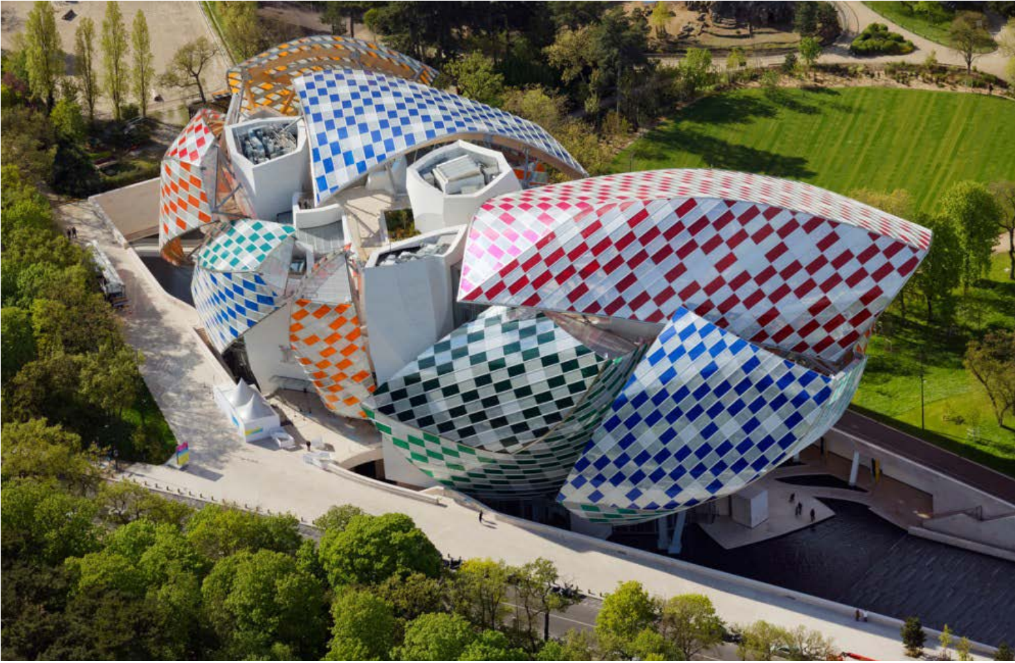
Architectural Outdoor - Louis Vuitton Fondatio, Paris, France
